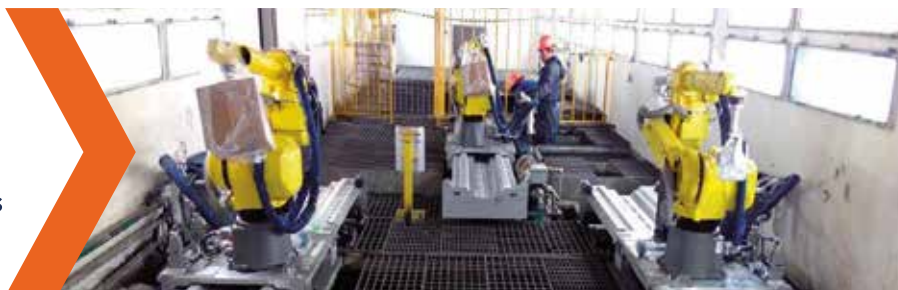
Installation of P250 robots NISSAN Aguascalientes
