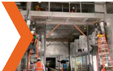
Installation of P700 robots in Agave project
