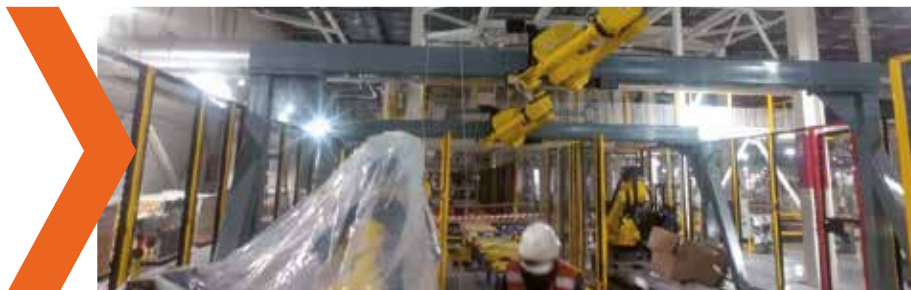
Installation of seal robots in Agave project
